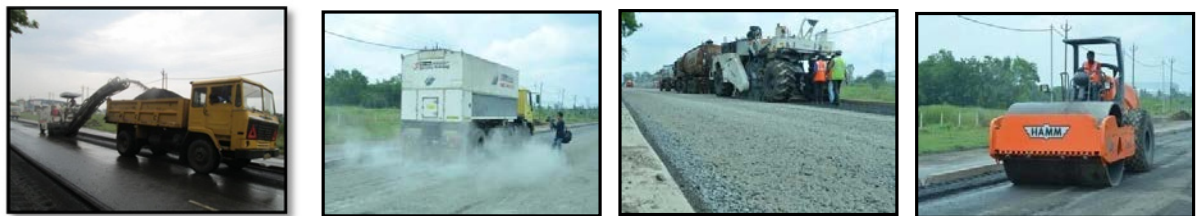
Fig.4. Photograph of Cold Recycle Construction in Progress
