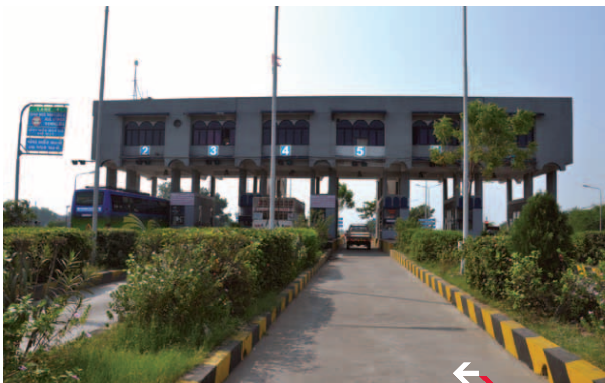
Vadodara Halol Toll Plaza
