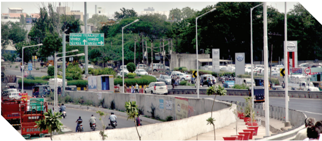
West Gujarat Expressway Limited (WGEL) Jetpur-Rajkot-Gondal Road
