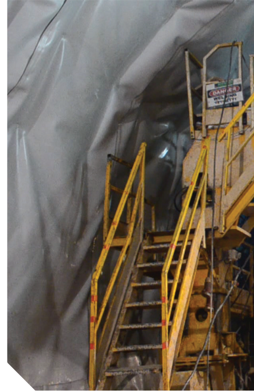
Waterproofing works in Chenani Nashri Tunnel
