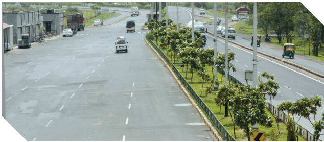
Gujarat Road and Infrastructure Company Limited (GRICL) Vadodara Halol Road
